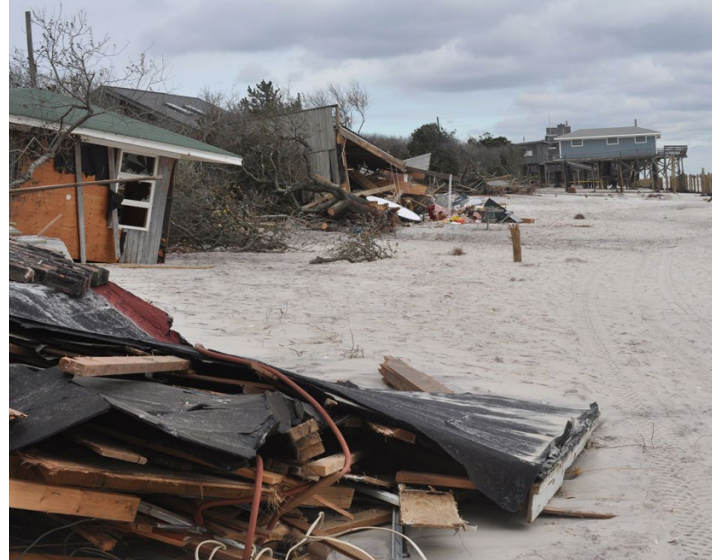
Hurricane Sandy destroyed or damaged many ocean front homes on Fire Island, NY. (Photo: Cheryl Hapke , USGS)
