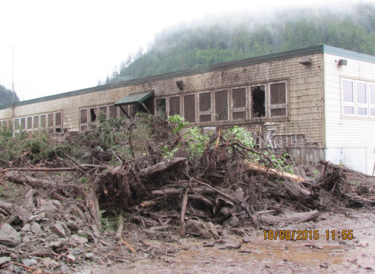
Photo 7 - damaged administration building at the Gary Paxton Industrial Park
