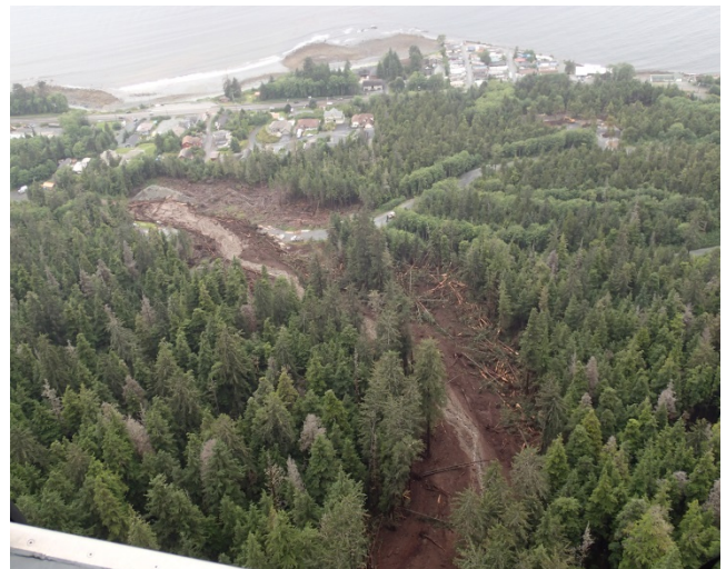
Photo 4 – Aerial view of Kramer Avenue debris flow. (Source: US Coast Guard)
