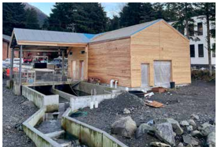
Construction almost complete on new spawning facility.
